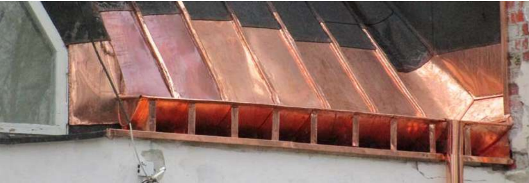
← The eaves on the eastern facade after a tentative reparation in November 2015. The aim was set to restore the form of the roof as well as to open a proper ventilation gap, which had been neglected in the earlier repairs as well as in the original construction. © The Imatra Parish/ Jari Nousiainen → A new copper lattice was added to North-Eastern corner to enhance ventilation under the copper-roof.
