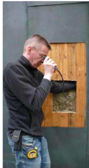
↑ Endoscopy of the roof structures by engineer Heikki Möttönen in May 2013.
